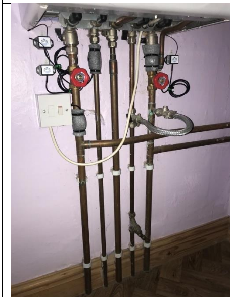
Pipework - pre meter install
